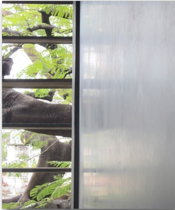
Figure 5.5. The chumum plaster wall at Golconde. Photo: Vijay Erasala.
