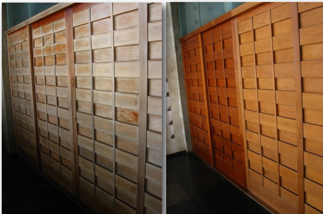
Figures 5.14 and 5.15: The teak doors before and then after sanding and some layers of shellac. Photos: author.
