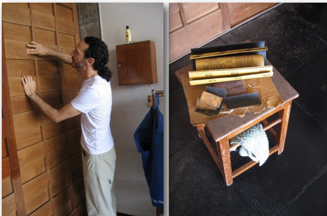
Figure 5.12 and 5.13: The author sanding the teak doors and the supplies used for the job. Photos: Sue Crothers and the author.
