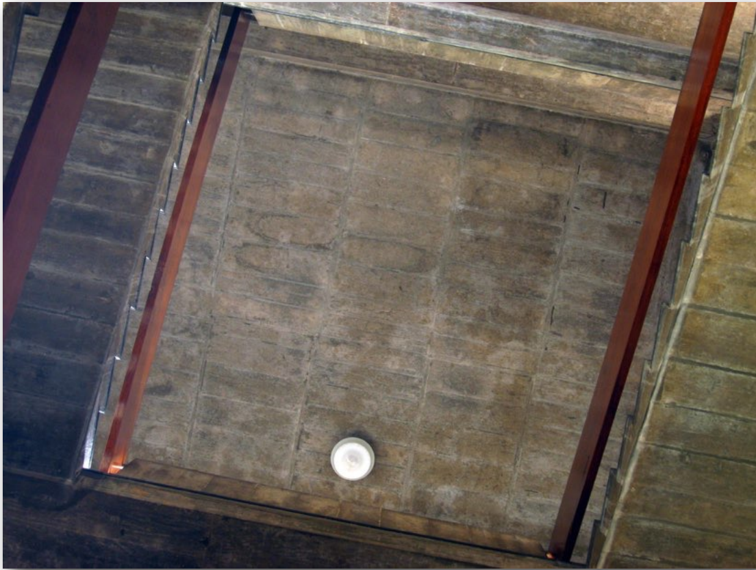
Figure 5.18. Golconde entrance looking up through the staircase to top floor ceiling, all made with rebar enforced concrete with teak guardrails. One can see the imprint of the wood grains from wooden formwork that molded the concrete. The surfaces were smoothed over with a carborundum (silicone carbide) stones. Photo by author.
